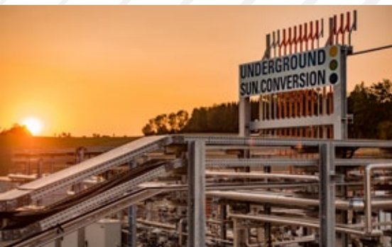
RAG-Anlage in Pilsbach/Oberösterreich Foto: RAG Austria AG/Karin Lohberger Photography
